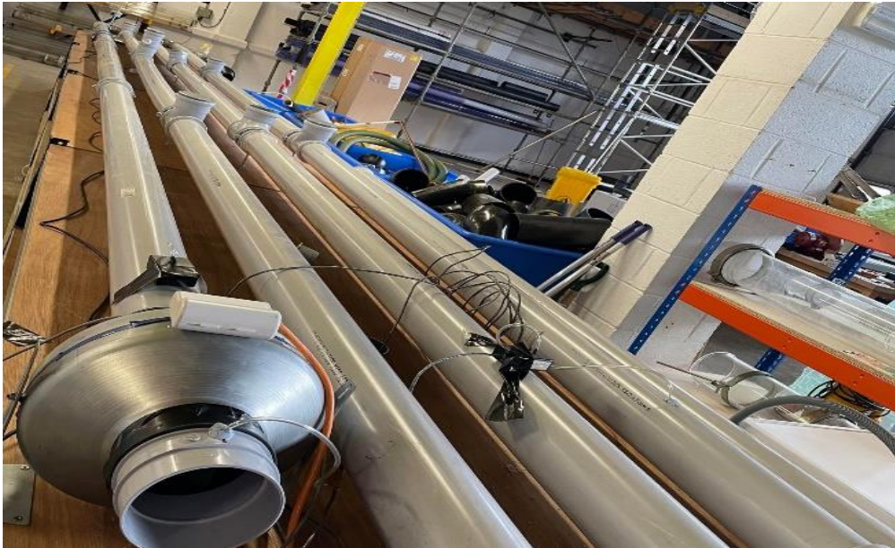
Figure 3 Laboratory test rig
