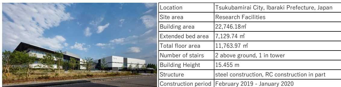
Figure 1 - Takasago Thermal Engineering Innovation Center
