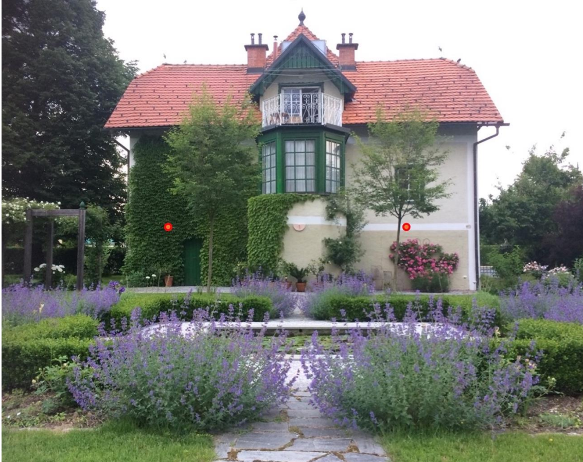
Figure 3 Green façade on the symmetrical house (position of sensors is marked with red dots)
